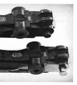
The Navy's solution to the toggle axle problem. The 1906 (top) has pin head diameter of 0.134"; the M1908 has head diameter of 0.360".
